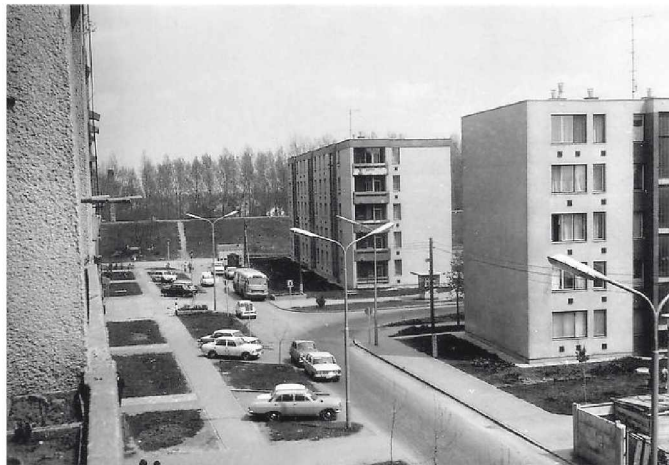
8. Table. Brick walling buildings in Szeged-Tarjánváros with the earliest bus terminal and the dam in the background
