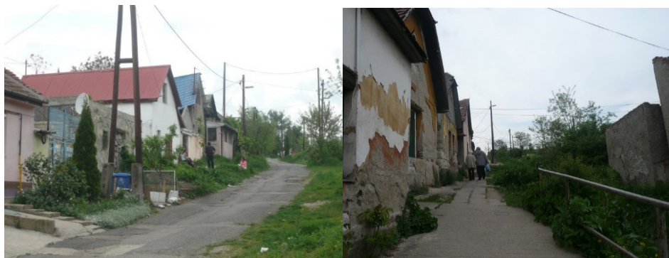
Photo 1: Neglected infrastructure and buildings
