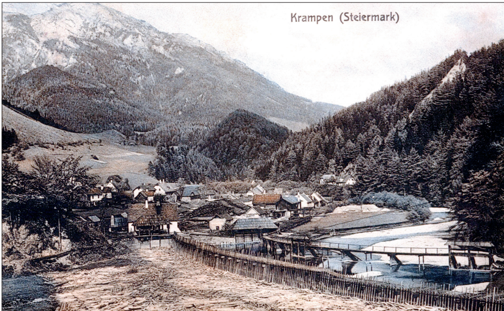
Figure 2 The Mürz rake at Krampen near Neuberg an der Mürz, built by the monastery of Neuberg an der Mürz, used until the 1950s (collection Reismann)
