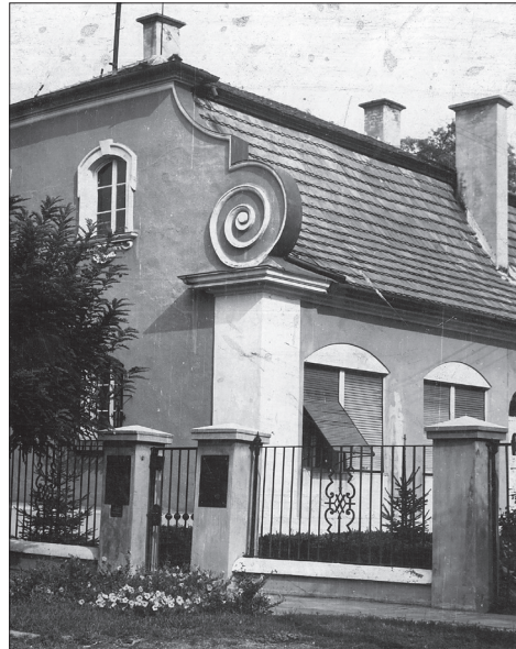
Figure 2 A front elevation volute of the Kner Villa (1925, architect: Lajos Kozma), shown in a photograph taken after the World War II
