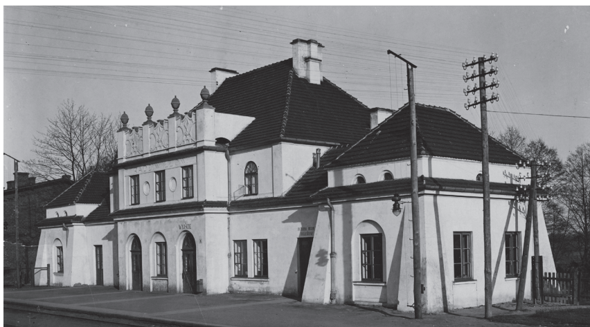
Figure 16 Radziwiłłów railway station
