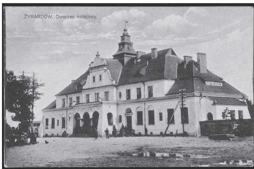
Figure 15 Żyrardów railway station
