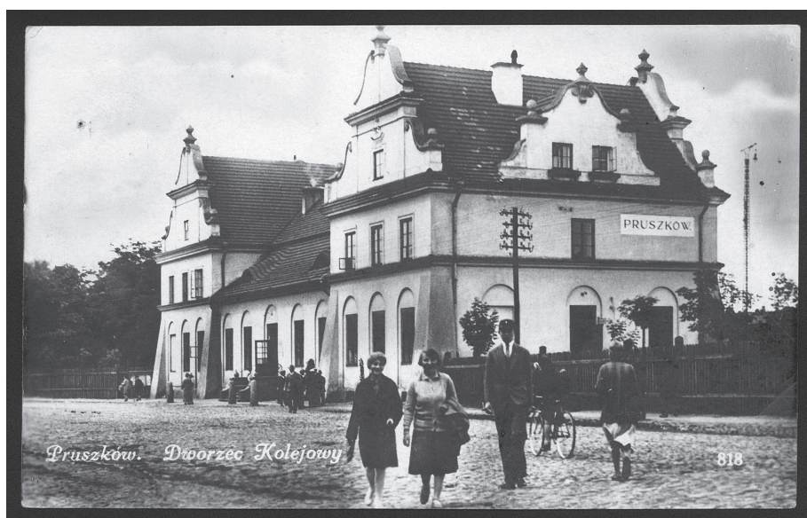
Figure 21 Pruszków railway station
