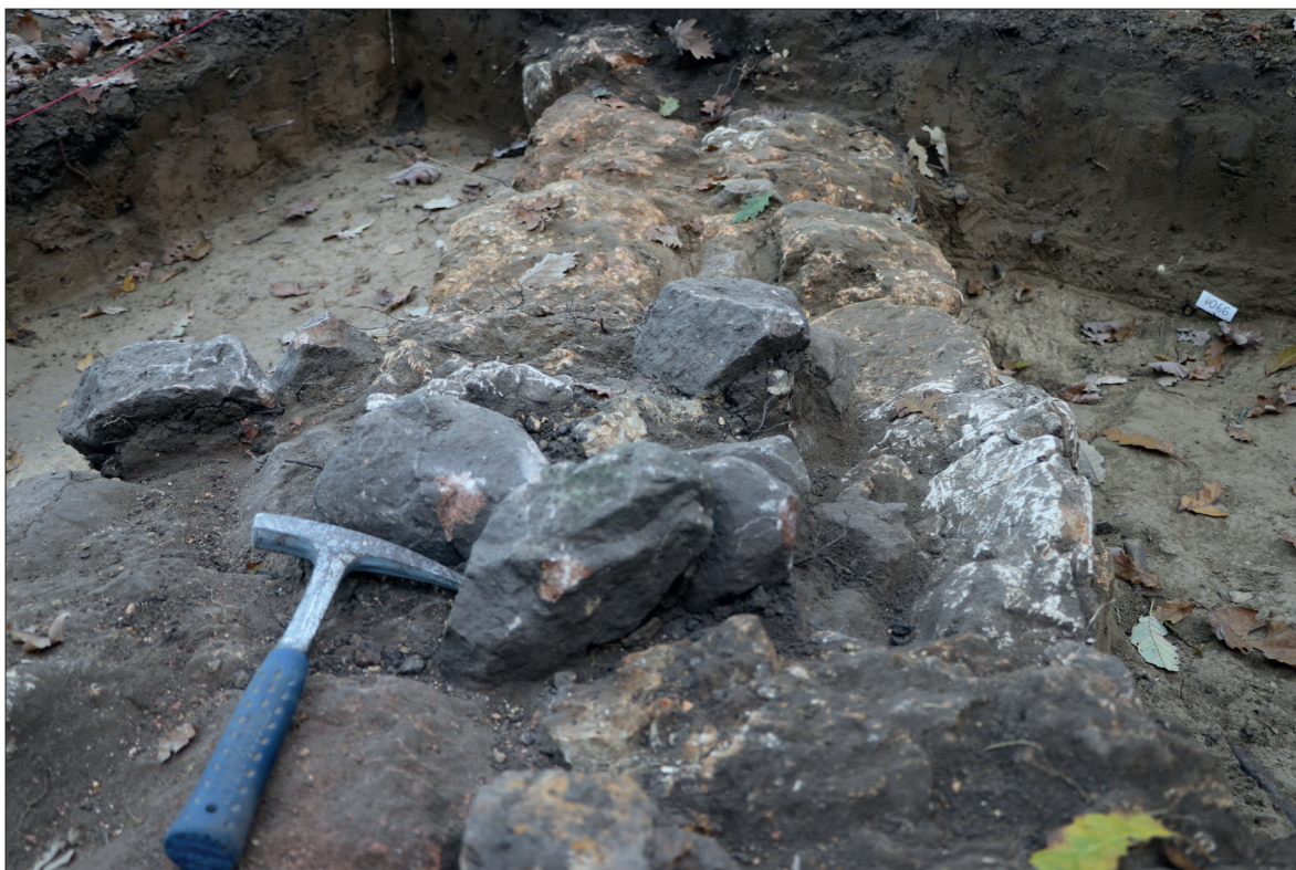
Fig. 3. Northern wall foundation of the excavated building in Quadrats 1–4. Top: two bottom courses of limestone (photo by B. Simon).
