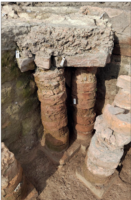
Fig. 11. In situ hypocaust pillars preserved in original height, and the pavement
