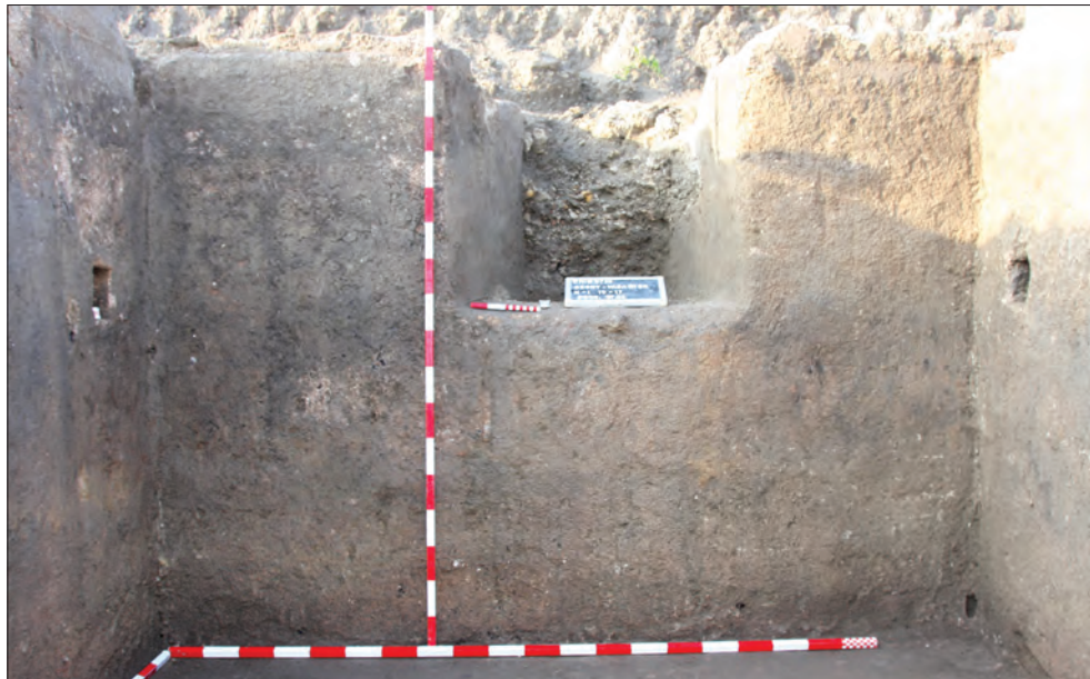
Fig. 70. The southern wall of Cellar 1 with a window (photo by L. Borhy)
