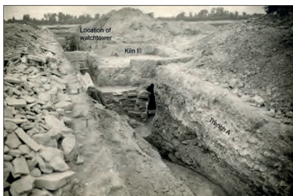
Fig. 7. Kiln I from the south
