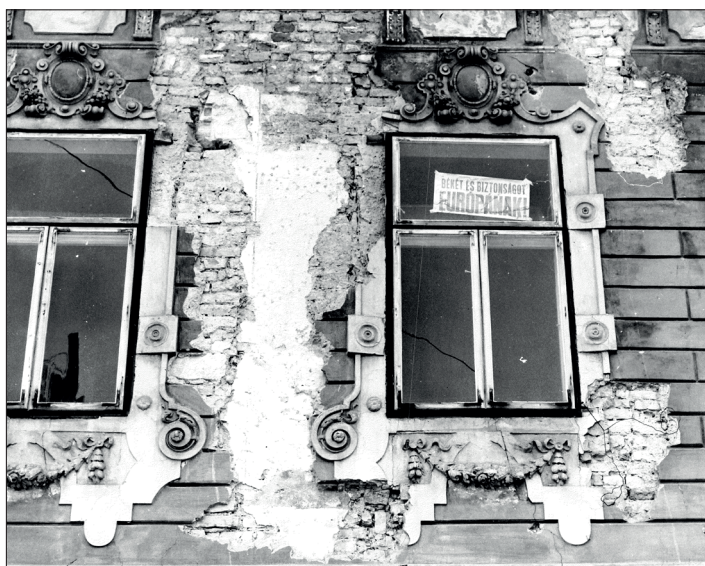
Fig. 3. Openings XXa and XXb with the painted plastered wall between them (Hungarian Museum of Architecture, Data Archive on Jász Street, Inv. no. 22629).
