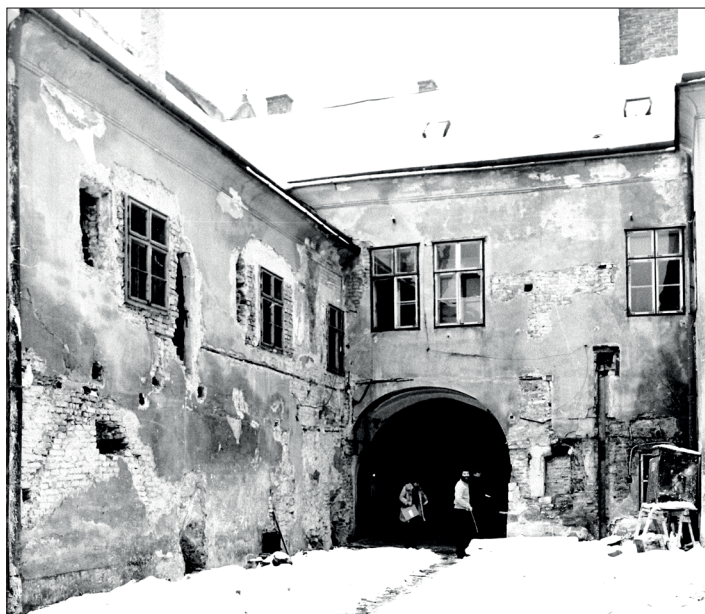
Fig. 2. Courtyard façade with the exposed medieval openings and other details (Hungarian Museum of Architecture, Data Archive on Jász Street, Inv. no. 22629).
