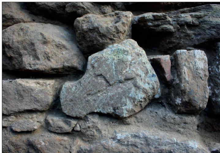
Fig. 8. A mediaeval vault rib in secondary position (photo: R. Rakonczay).
