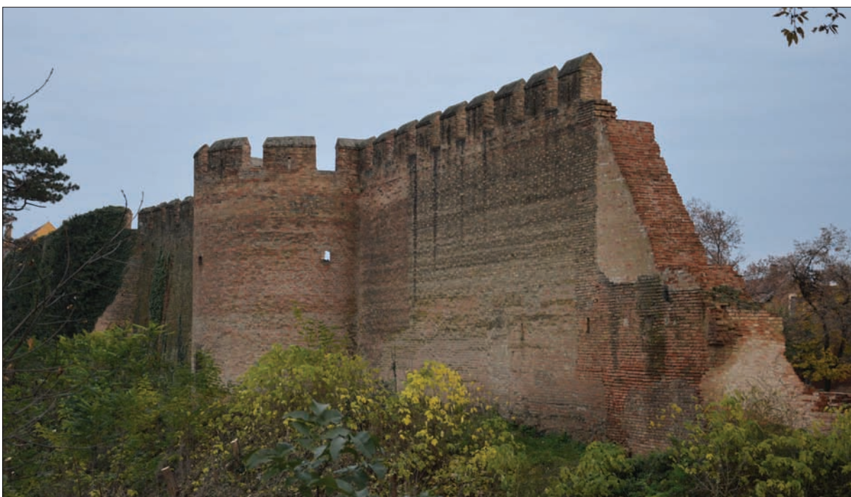
Fig. 28. Crenellated mural tower of the northern wall of Újlak uppertown (The battlement did not preserve its original medieval form.).
