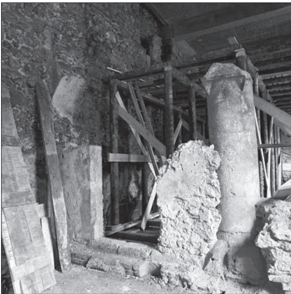
Fig. 8. In situ stone pillar in the longitudinal axis of the western great hall at Várpalota Castle (Photo of A. Gergelyffy from 1976, Hungarian Museum of Architecture and Monument Protection Documentation Centre, Photo Repository).
