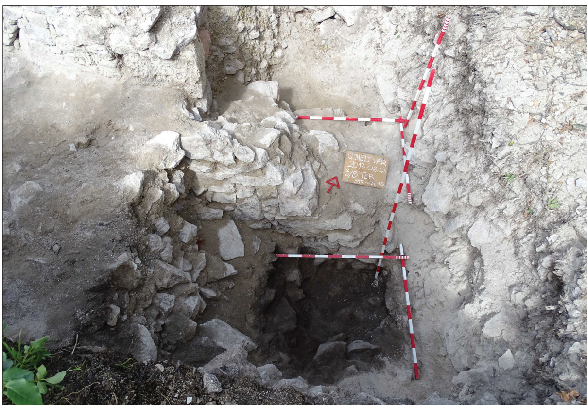
Fig. 3. The buttress used to support the merging of the tower's southeast corner and the connecting eastern castle wall.
