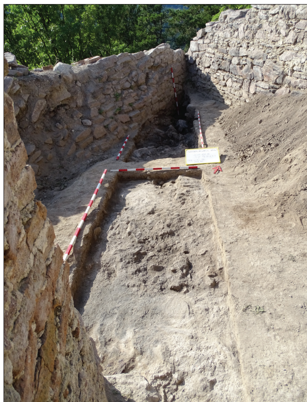
Fig. 8. The cross-section of the ground floor of the tower and the remains of the earlier ground floors.
