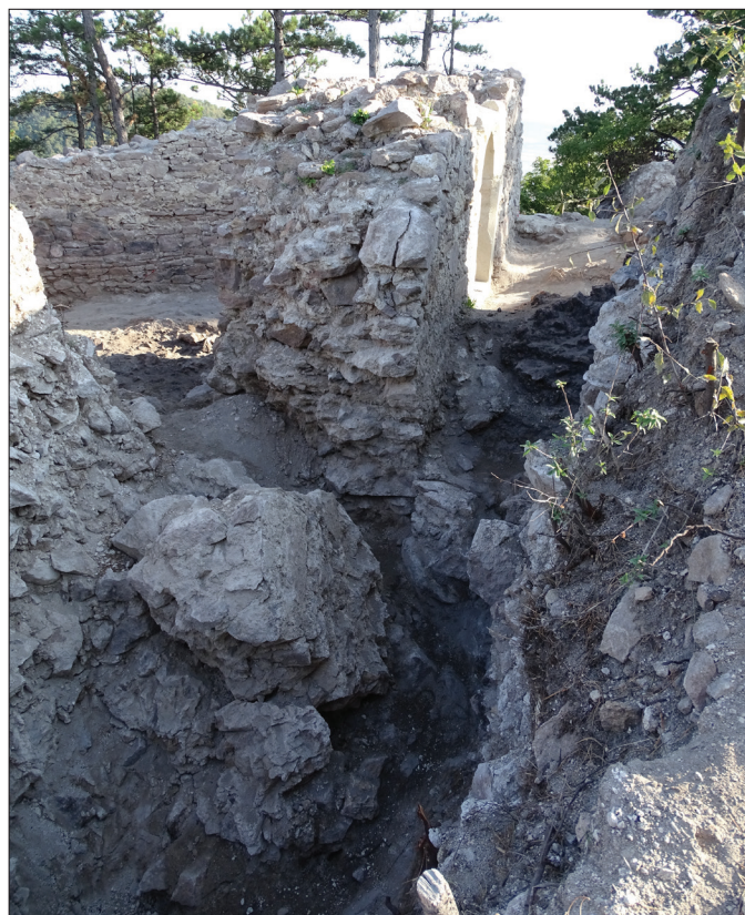
Fig. 7. The fallen southwestern corner of the triangle-shaped tower.
