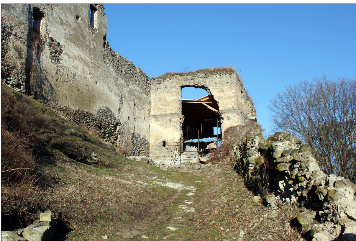
Fig. 2. View of the gate tower from south (30. 12. 2016).
