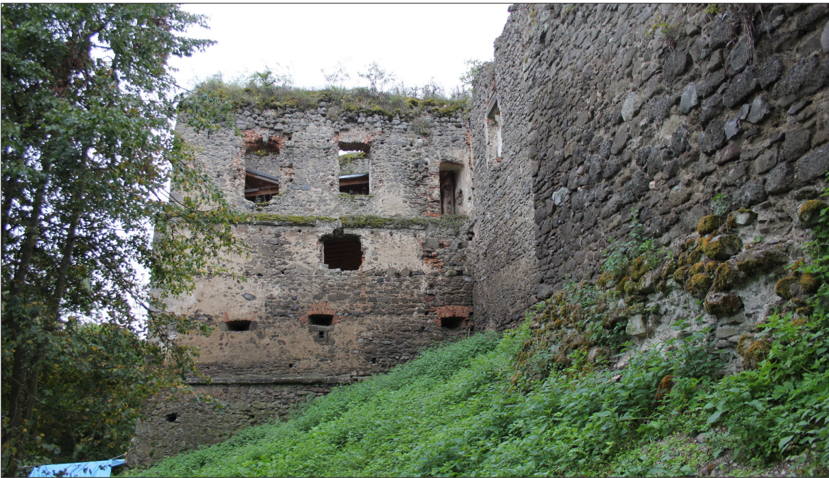
Fig. 3. View of the gate tower from north (10. 08. 2016).
