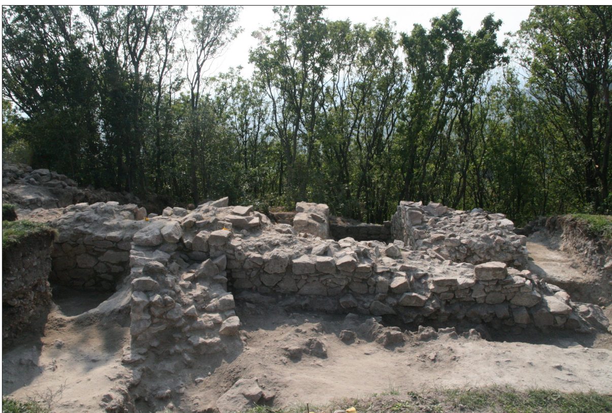
Fig. 13. The eastern wall of the building connected to the western wall of the castle (Photo: Dóra Hegyi).
