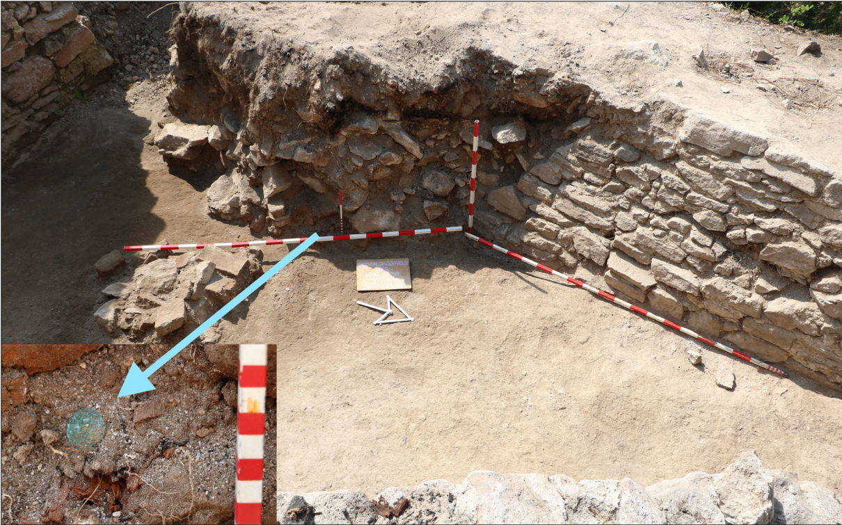
Fig. 4. The cleaning of the tower and the demolished western wall of it.
