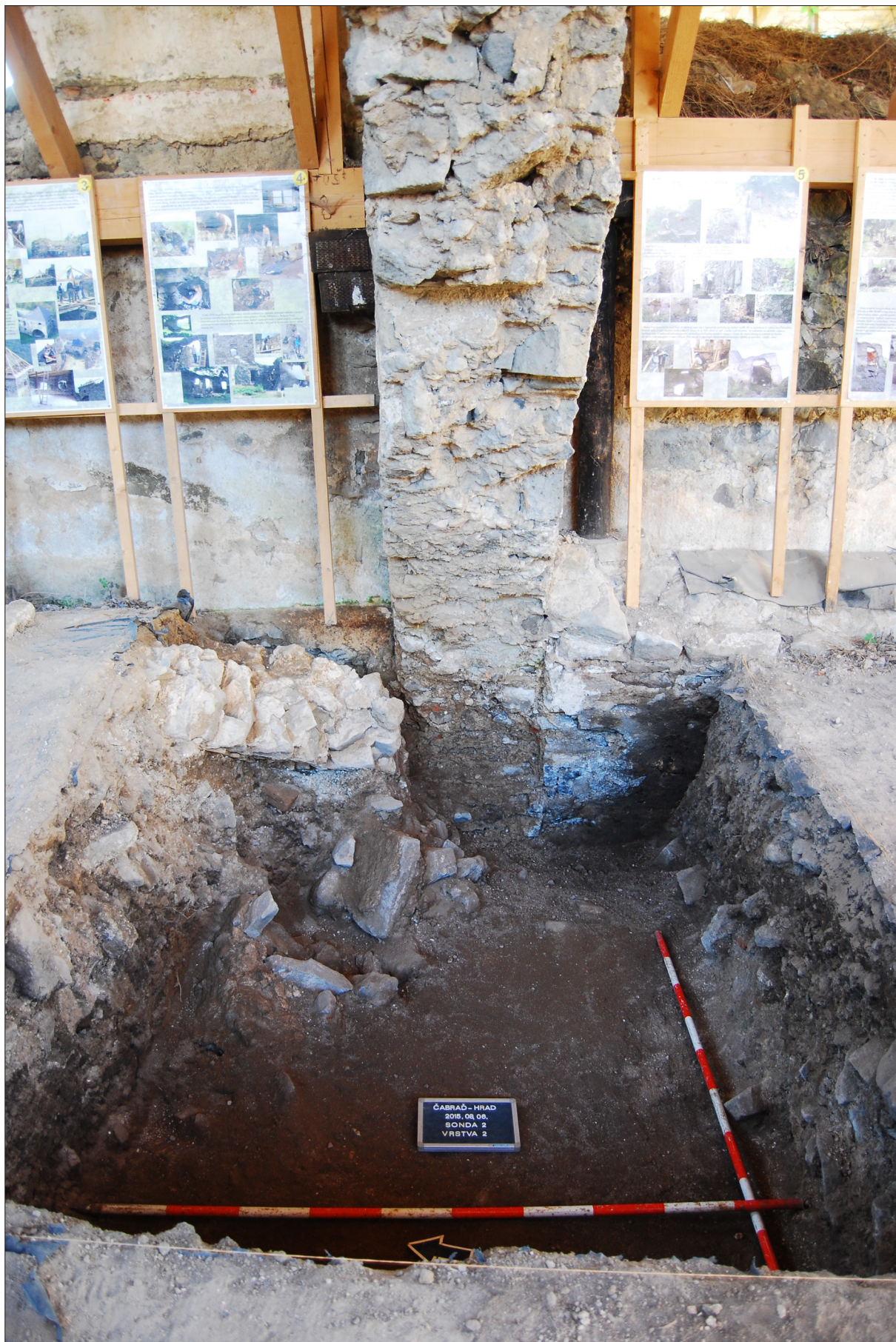
Fig. 17. The northern partition wall in the tower with no traces of the foundations (Čabrad).
