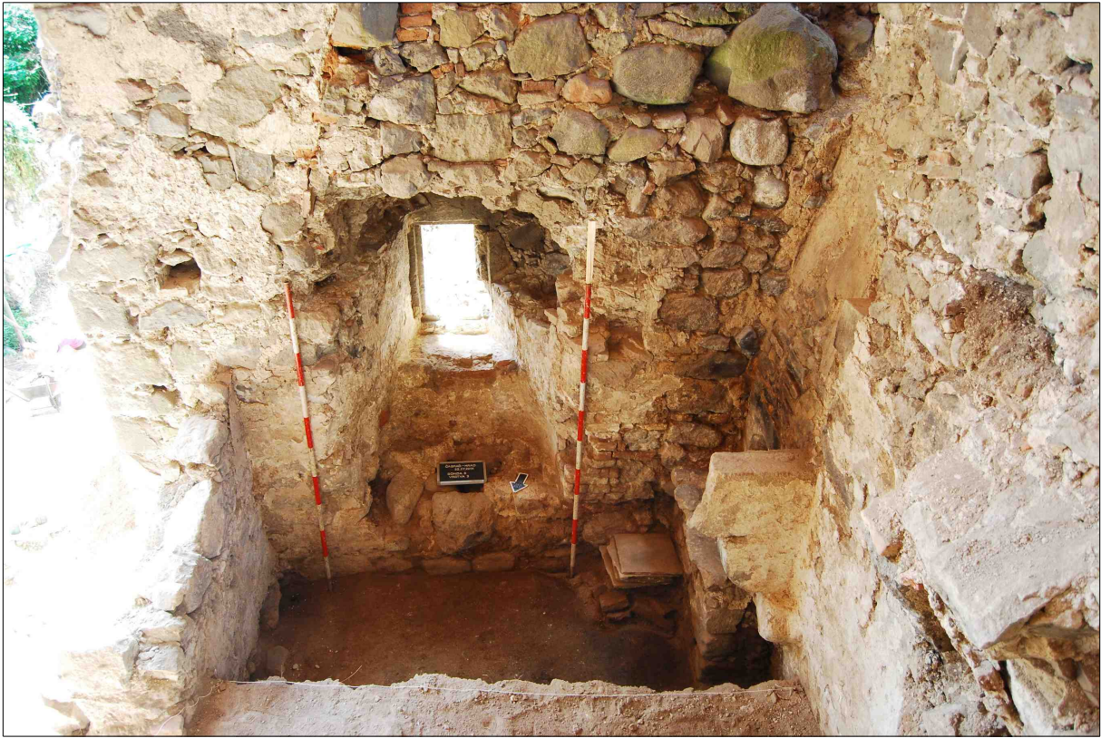
Fig. 8. Window in the southwestern corner of the tower.
