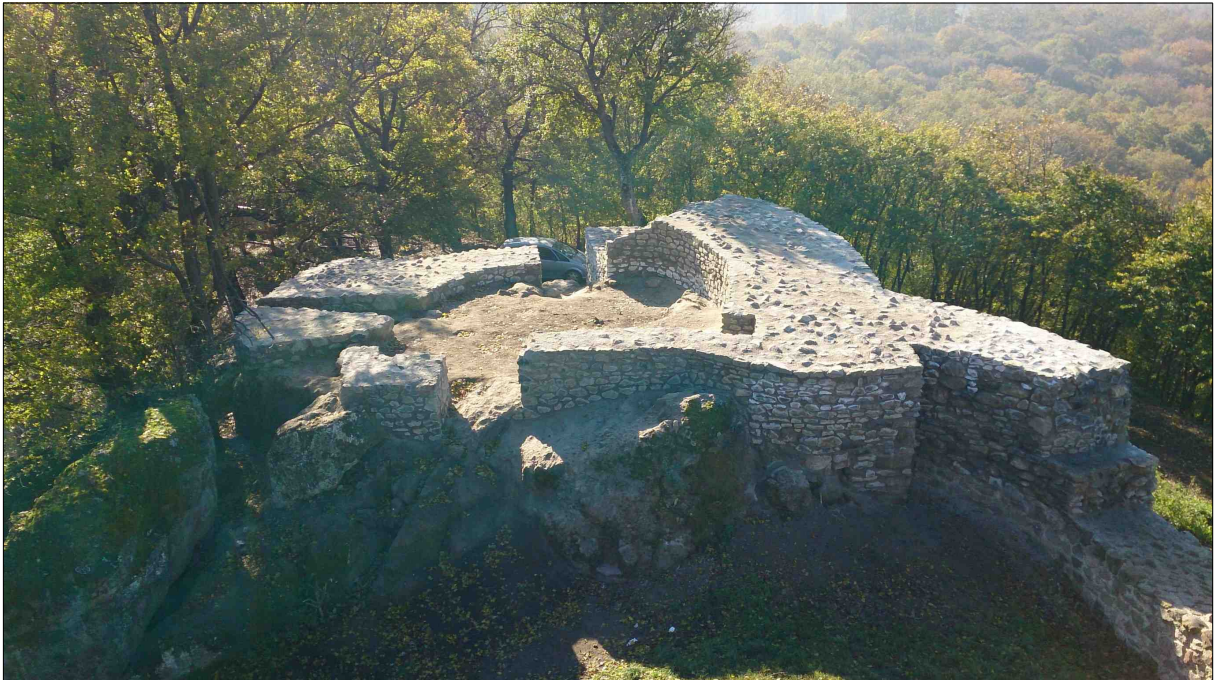
Fig. 15. Partially reconstructed tower in November 2014 (Photo: Péter István).
