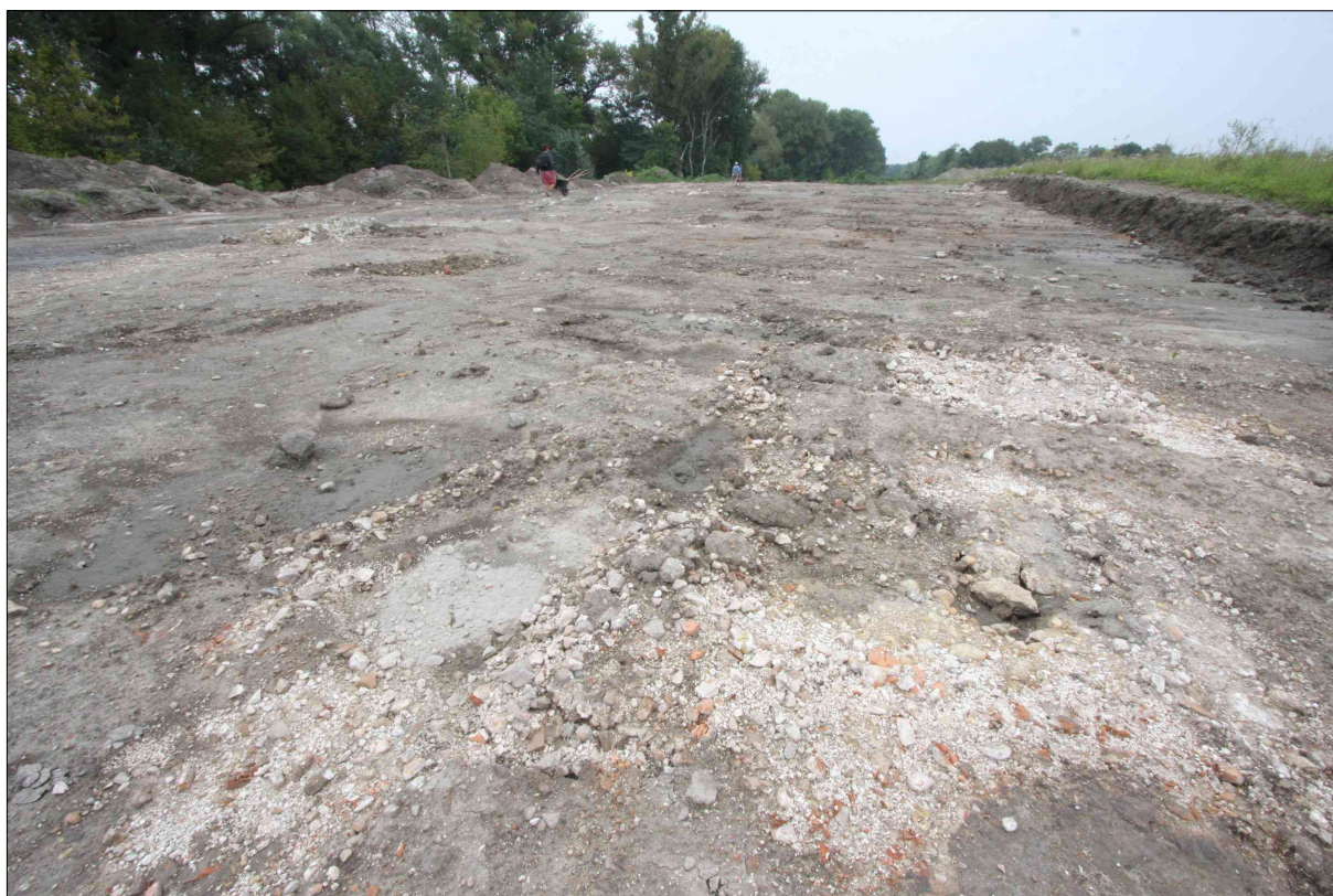
Fig. 3. The site after the removal of topsoil.
