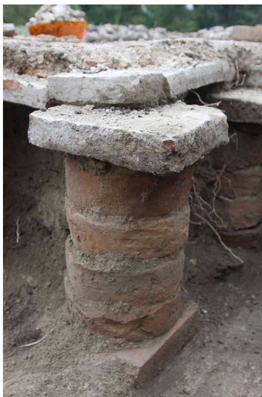
Fig. 12. Pilae stacks from the bath.
