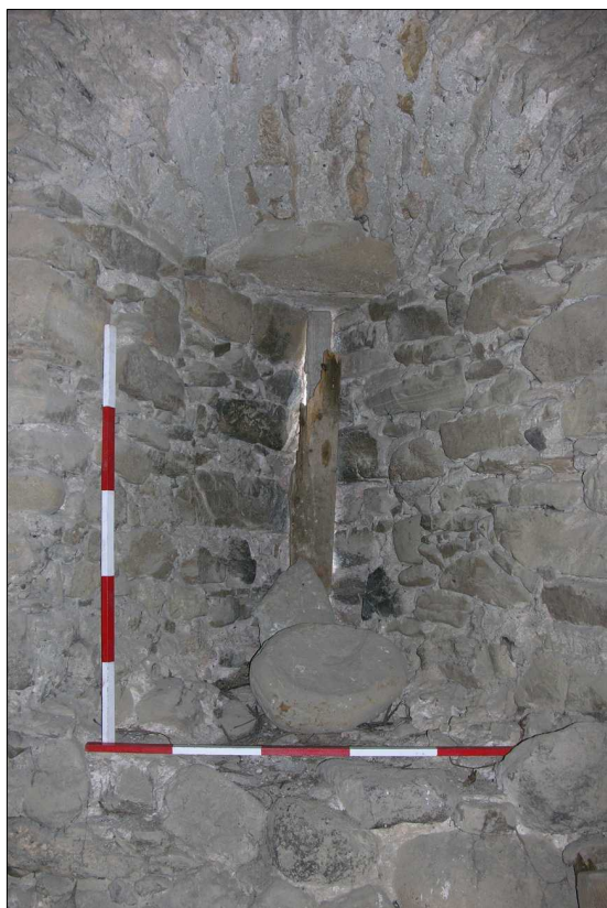
Fig. 18. Loopholes at Crăciunești church-tower, second floor, north side (Photo: A. Sófalvi).
