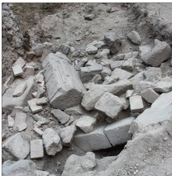
Fig. 23. The fallen fragments of the gate in the second trench (Čabrad).
