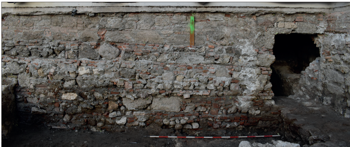
Fig. 28. Foundation wall of the eastern wing (photo: ArchaeoProtect Ltd.).
