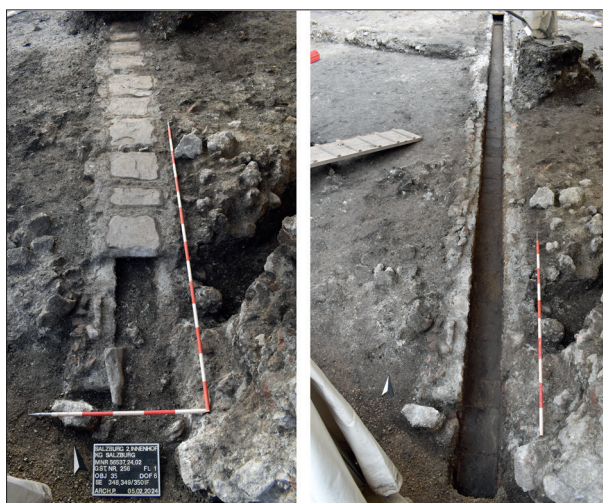
Fig. 37. Remains of an 18th-century sewer (photo: ArchaeoProtect Ltd.).
