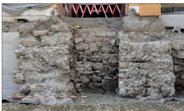
Fig. 29. The massive buttresses, which support the weight of the ground-floor arcades (photo: ArchaeoProtect Ltd.).
