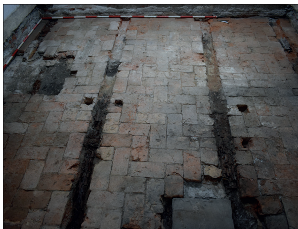
Fig. 36. Foundation of the brick floors from the 18th century (photo: ArchaeoProtect Ltd.).
