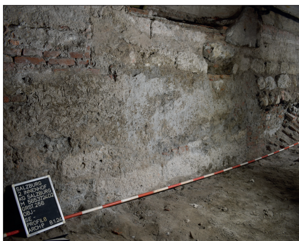
Fig. 30. The original walls of the 16th-century cellar (photo: ArchaeoProtect Ltd.).
