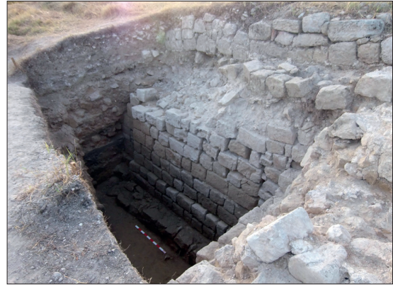
Fig. 25. Superposition of the late antique and medieval defensive walls (photo by V. Varbanov).
