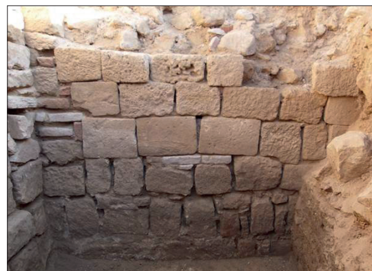
Fig. 24. Outer face of the late antique tower (photo by V. Varbanov).
