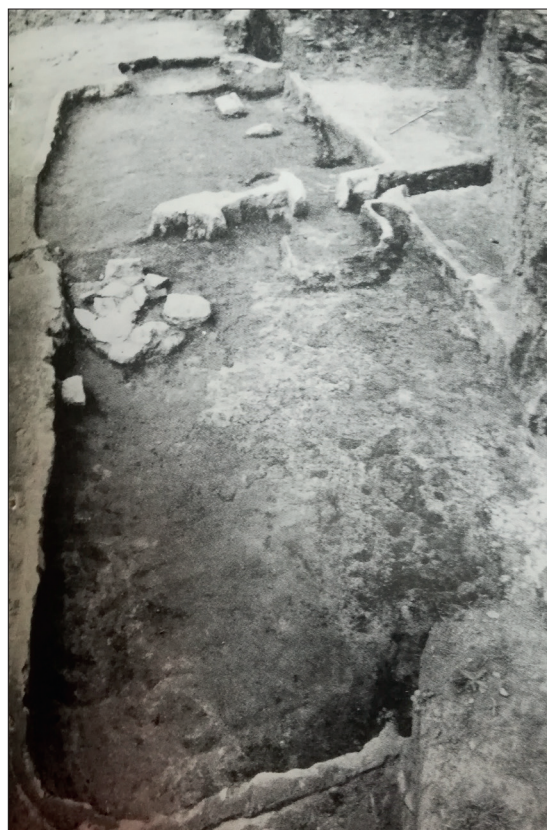
Fig. 3. Medieval dwelling with two rooms in fort of Yatrus (after DIMOVA 1975).
